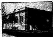
Typical Repeater Station
