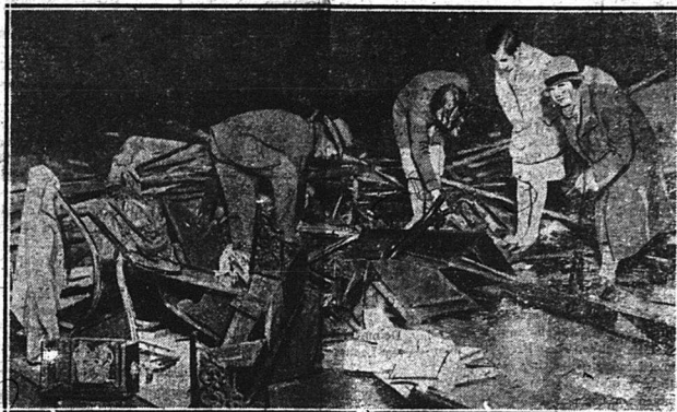
Ruins of a school at La Plata, Md., were searched after a cyclone leveled the building, crushing out the lives of thirteen pupils.
